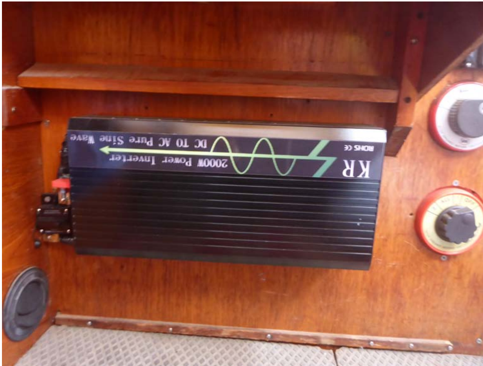
Figure 37 DC to 220 V converter. The automatic 150A fuse is seen to the left.
