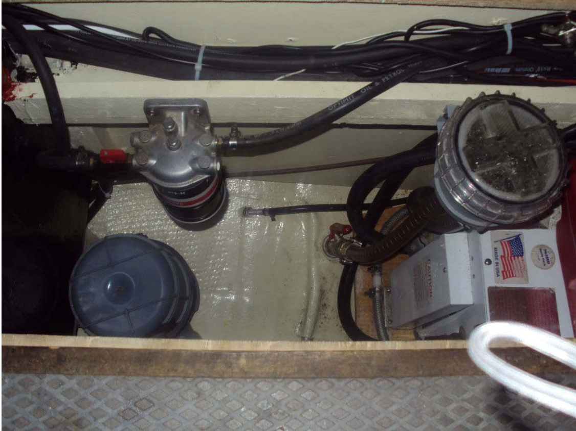
Figure 22 Bottom left of motor room. Top left shows the diesel filter and water separator, bottom left the water lock and silencer, top right the water filter, in the middle right the inlet water valve (red handle) and to the right the hot water tank. The small hose in the middle leaving to the right is a tube containing the cable for the log.
