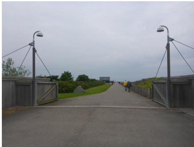
Gates which are closed in case of storm
