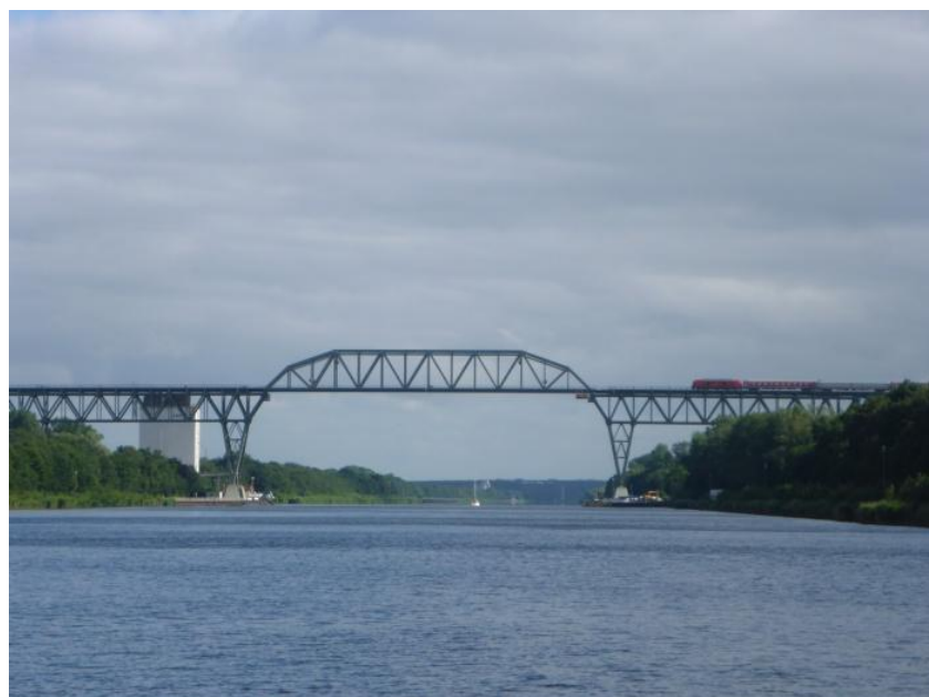
A railway bridge
