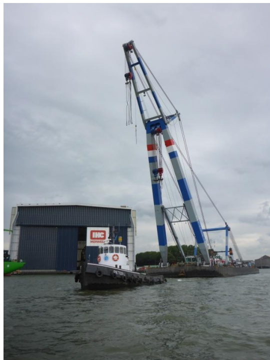
The crane stops
