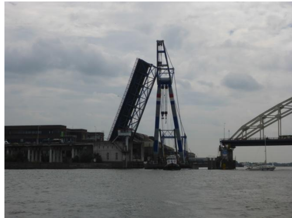
Second bridge. The crane is passing
