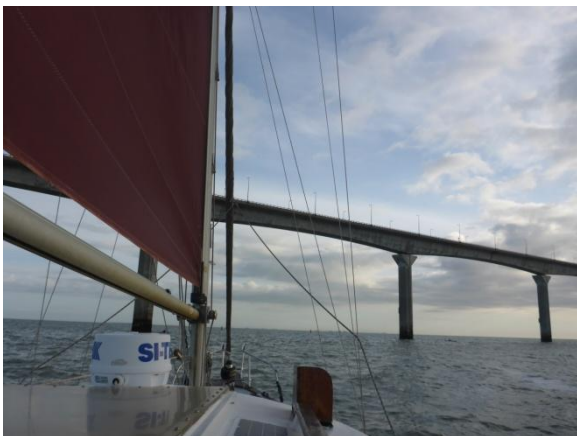
We pass under Ile de Ré bridge
