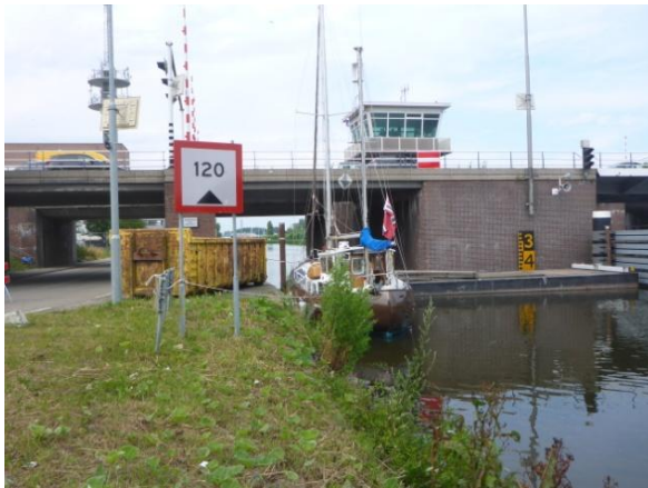
The bridge under repairs ...
