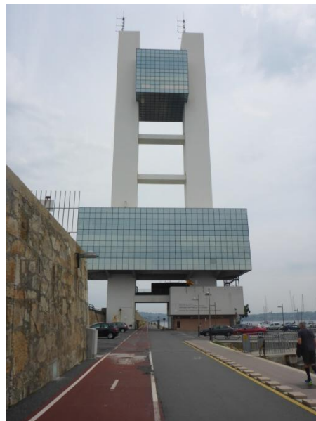
The tower on the jetty
