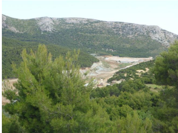
A dam under construction
