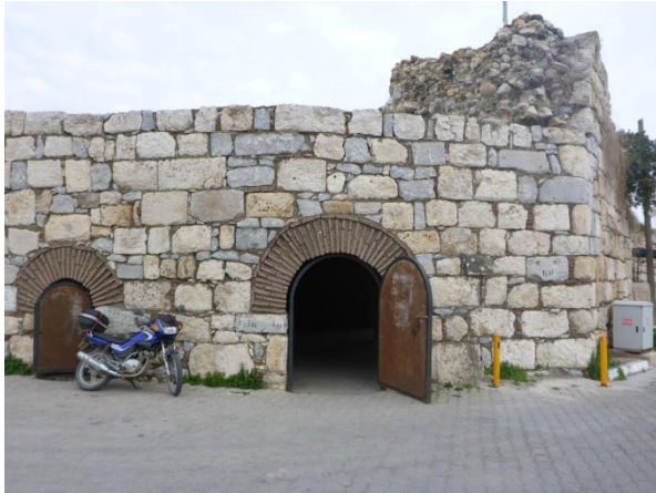
The wall. Outside ...
