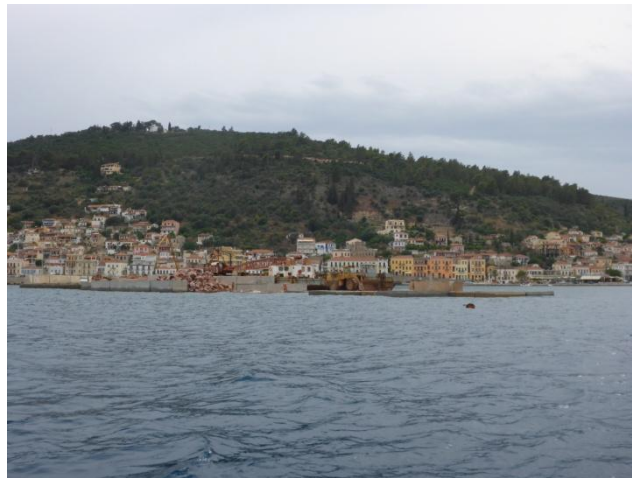
The jetty is under work
