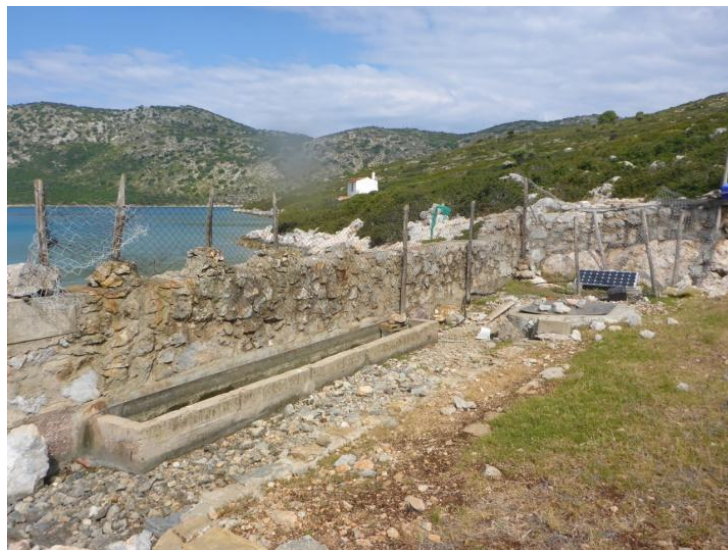
The water basin alimented by solar panel
