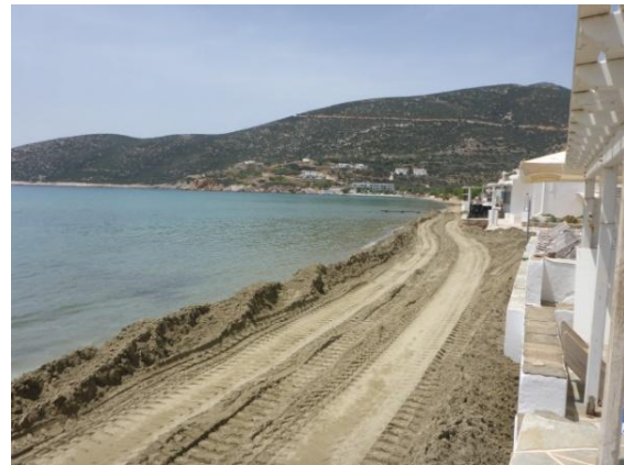
Work on the beach
