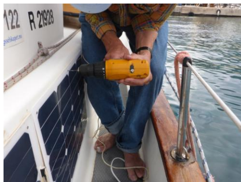
Jens changes a solar panel
