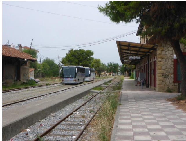
The old train station, now a bus station
