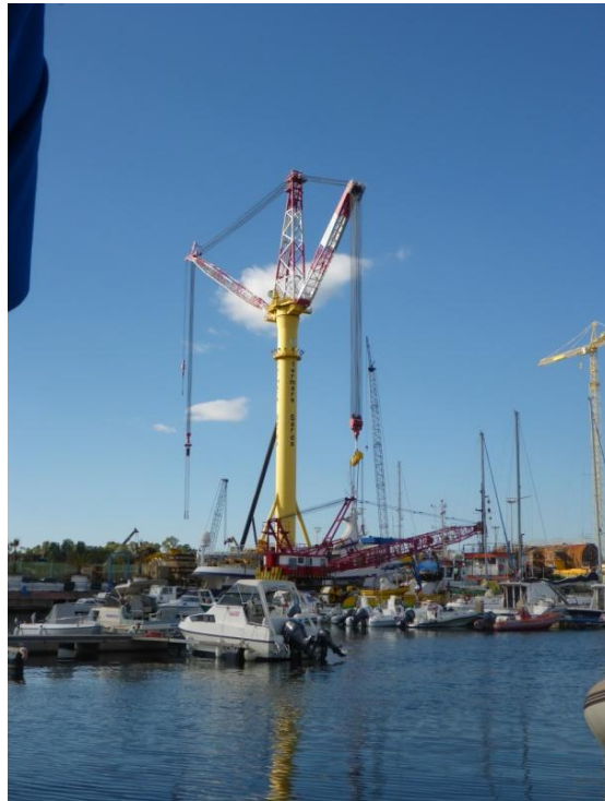
The huge crane in Arbatax harbor
