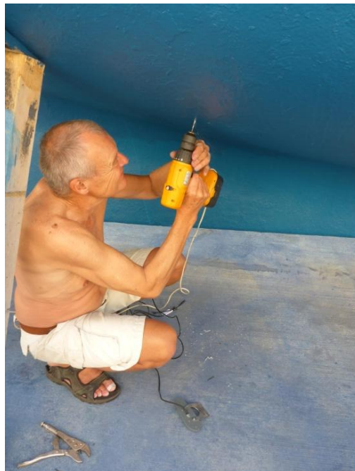
Jens installs a new deep sounder
