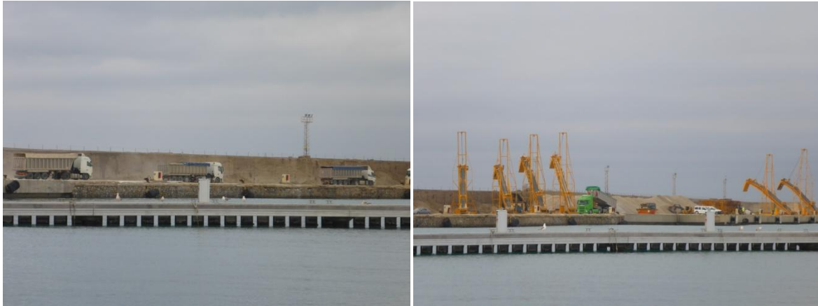
Trucks and excavators on the dike
