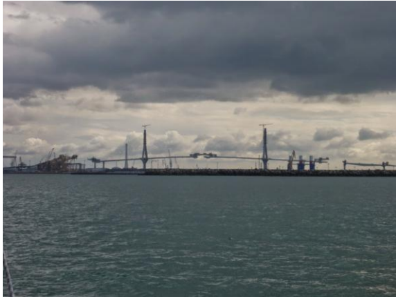
The bridge under construction
