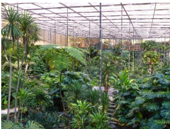
The cold greenhouse
