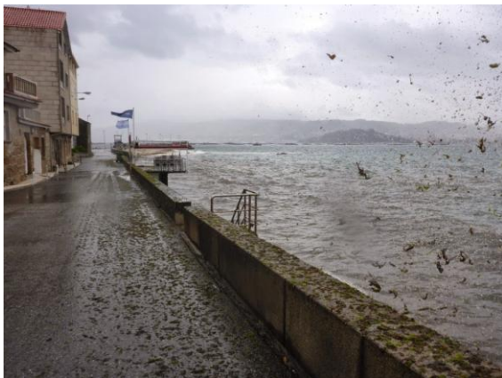
The waves are passing over the wall
