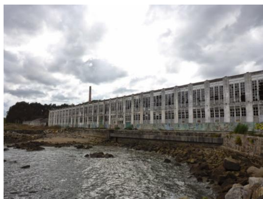
The whale's treatment plant
