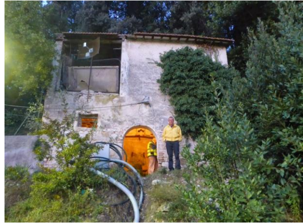
The abandoned house
