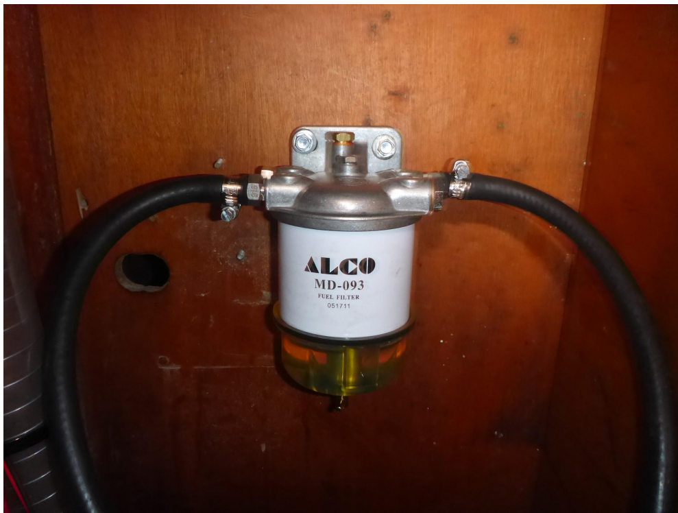
Diesel pre-filter, under the stairs.
