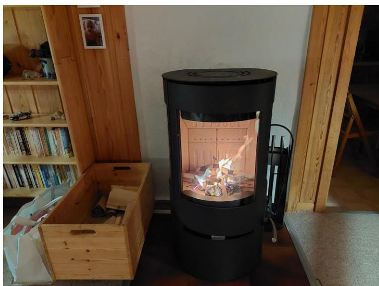
We finally installed a new wood stove, ready for the winter.
