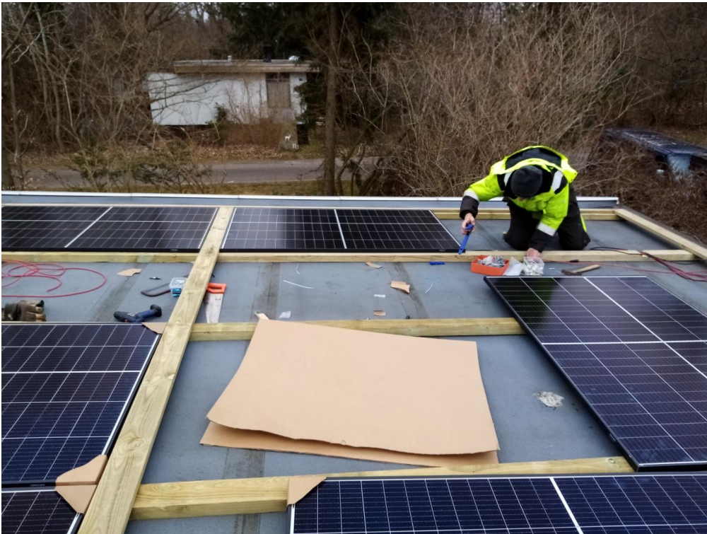
Jens installs solar panels at our house in Denmark
